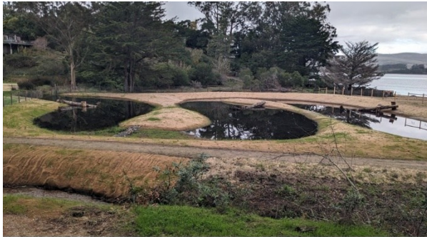
Chicken Ranch Beach Wetland Restoration after grading Photo by Tom Gaman
