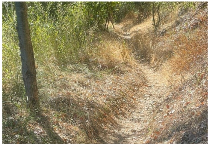
Concrete Pipeline Trail trench forming by David Long
