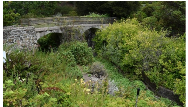
Bridge across Wildcat Creek, Regional Parks Botanic Garden, in Tilden Park - Berkeley CA Photo by Richard A Walker © Creative Commons 2020
