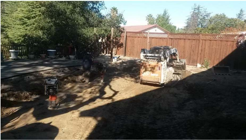
<- Backyard being graded in (defunct) pool area. Photo by Stacey Pogorzelski
